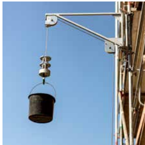
Scaffold swing arm
